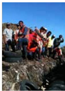
Leachate drainage by used tires
