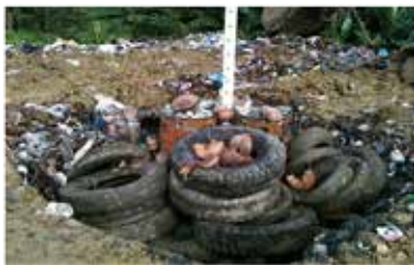
Used tires are buried around the drums in order for the facility not to be damaged by machines' daily operation.
