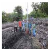
3) Installation of gas venting pipe
