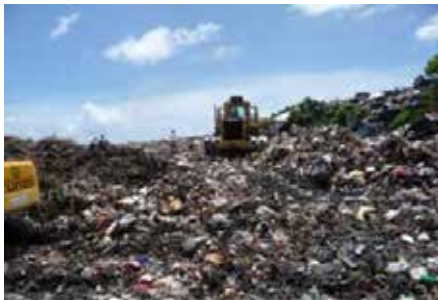
Access road, before work
