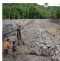
2) Reusing waste tires for an approach road
