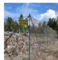
4) Installation of fence and sign boards
