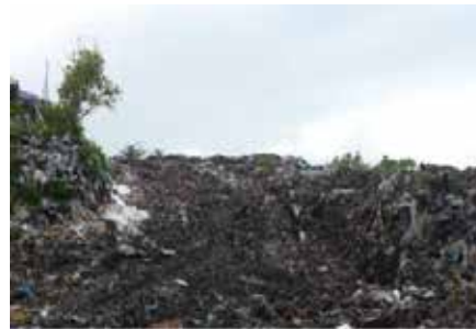
Access road, after work
