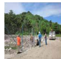
After (inside dumpsite)
